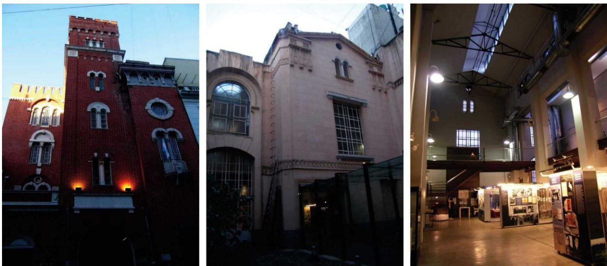
Fig. 10, 11,12. Usina Montevideo reconvertida en Museo del Holocausto / Montevideo power station reconverted as Holocaust Museum (Dujovne, Hirsch & Grinberg, Dwek, Sartorio, Iglesias, 1999-2000). (fotos/photos: Carolina Quiroga)
